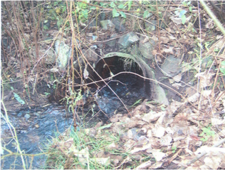
2- 15" CMP pipes under Rapp Road
